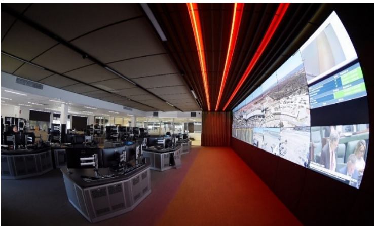
Airport Control Centre
