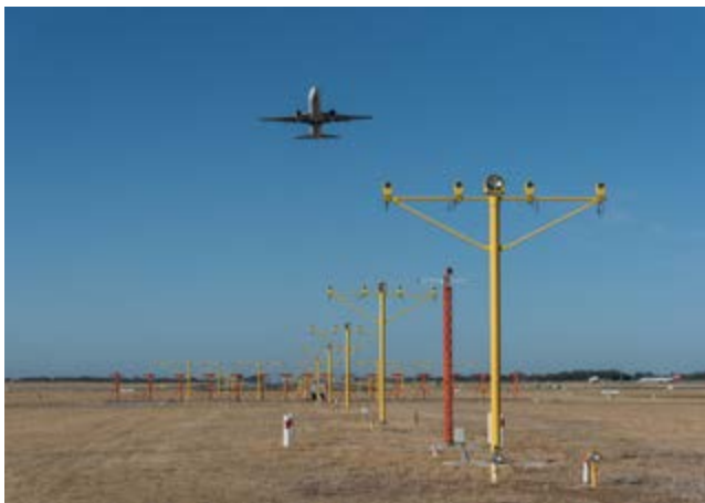
Figure 16-8 High Intensity Approach Lighting at Perth Airport Example Source: Perth Airport
