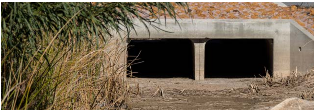
Figure 16-10 Example drainage outlet Source: Perth Airport
